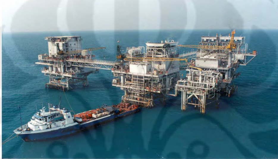
Gambar 3.1 Area Kerja Mike-Mike Flow Station
