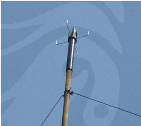
Gambar 3.4 E.F Lightning Terminal 1
