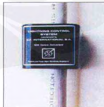
Gambar 2.25 E.F Lightning Counter
