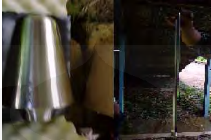
Gambar 2.26 Skylance Lightning Terminal dan Fibreglass Mounting
