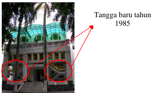
Gambar4. 1 Analisis Tangga Terhadap Façade Masjid Cut Meutia
