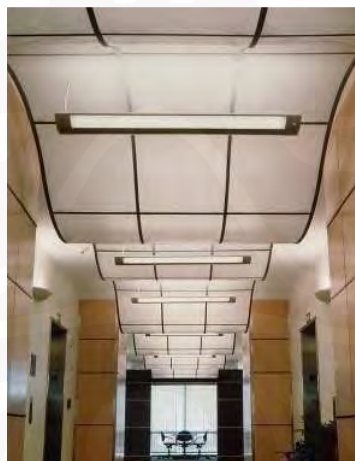
Gambar 3. 25 Luminous Ceiling
