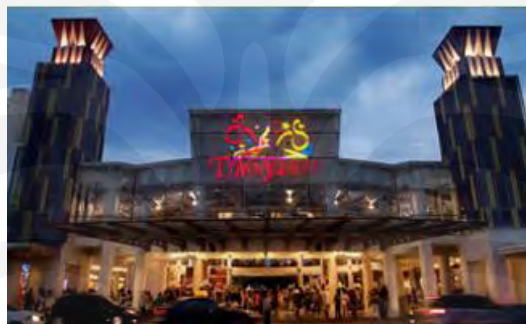
Gambar 3.15 Entrance Cilandak Town Square Sumber : http://www.townsquare.co.id
