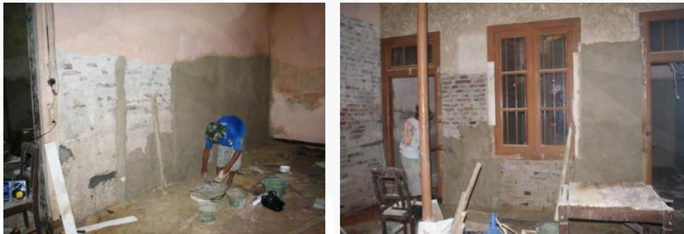
**Gambar 3.55 Plaster Ulang Pada Bagian Dinding Yang Dikupas**
