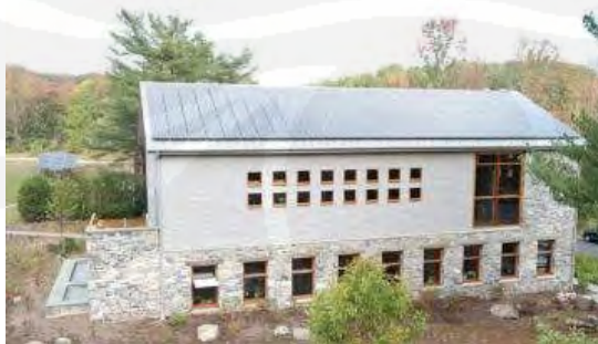
Gambar 3.57 Atap Willow School menggunakan stainless steel (Sumber. Bdcnetwork.com)
