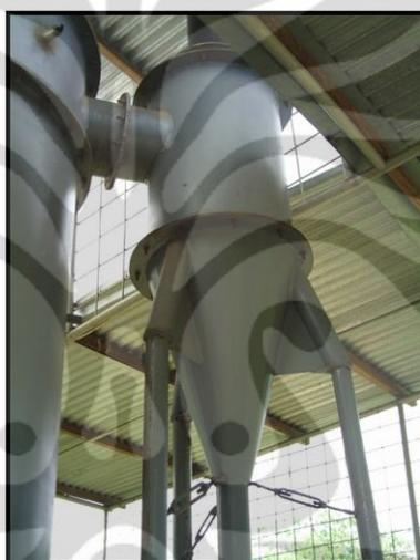
Gambar 2.17 *Cyclone Separator Fluidized Bed Combustor* UI
