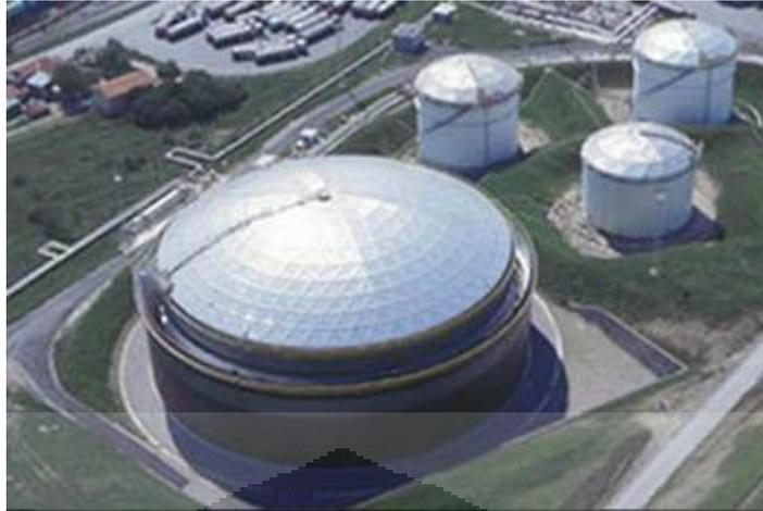
Gambar 2. 5 Contoh *dome roof tank*
