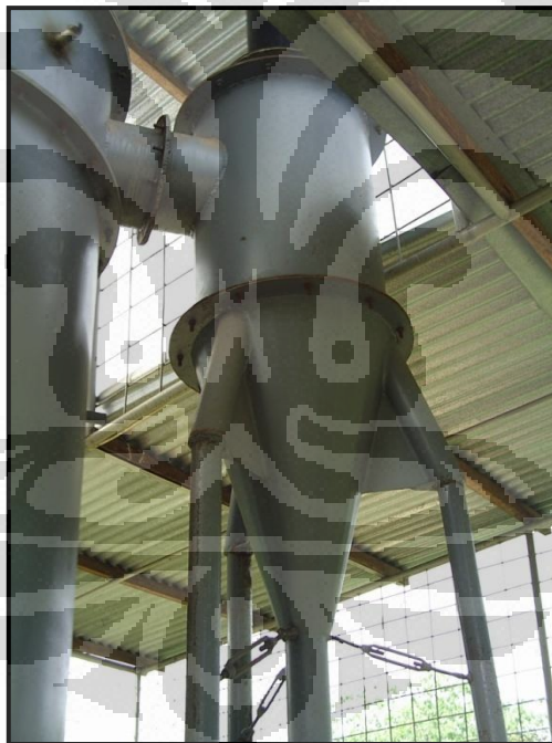
Gambar 2.17 Cyclone Separator Fluidized Bed Combustor UI
