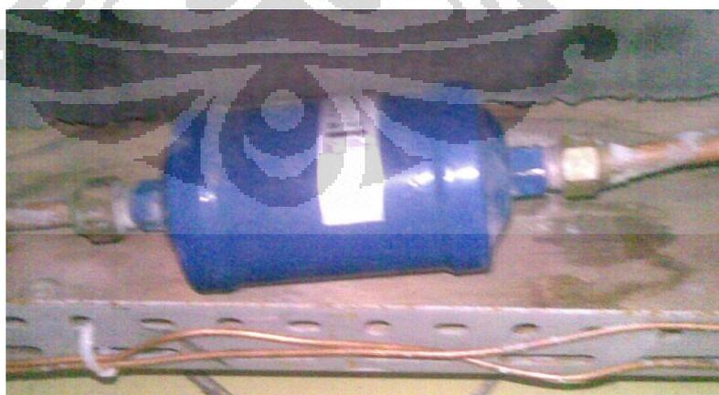
*Gambar 3.11. Liquide line filter drier*
