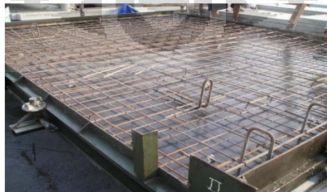
Gambar 4.13 Pembesian Panel Facade
