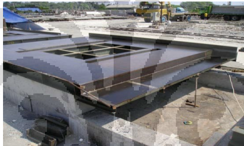
Gambar 4.12 Moulding Panel Facade
