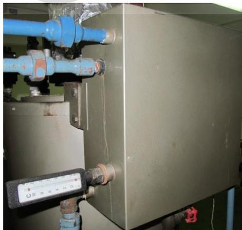
Gambar 3.10. Feed Water Tank
