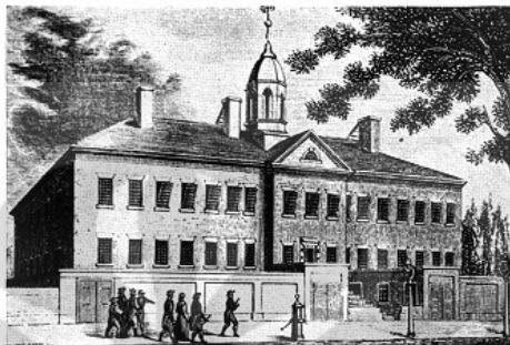
Walnut Street Jail, southeast corner, Sixth and Walnut Sts.
