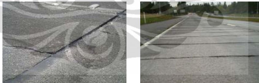
Gambar 2.6 Faulting
