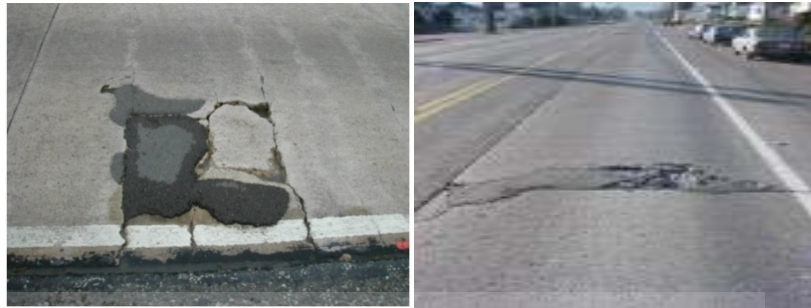
Gambar 2.17 Spalling
