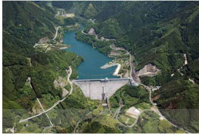
Figure 2.13. Kyuragi Dam (Takeo Office of River, 2008)
