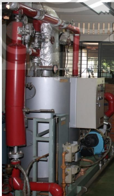
Gambar 3.5. Superheater
