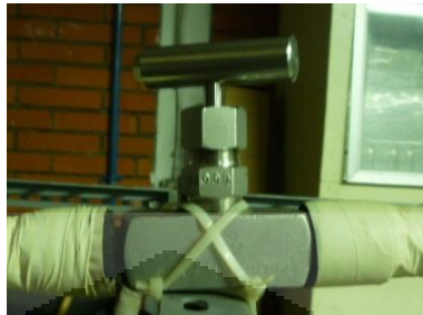
Gambar 3.6 Needle Valve
