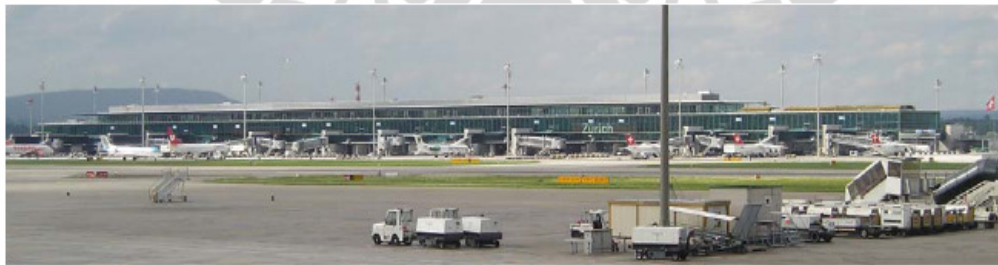
Figure 2.10 The Dock Midfield Zürich Airport
