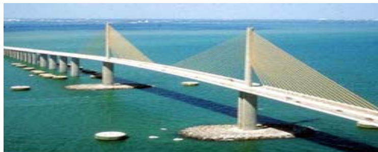
Gambar 2.2 Jembatan Cable-Stayed Sun Sky
