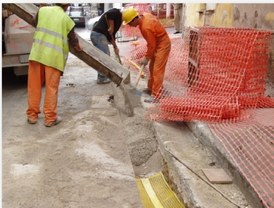
Figure 1.1. Backfilling Trench
