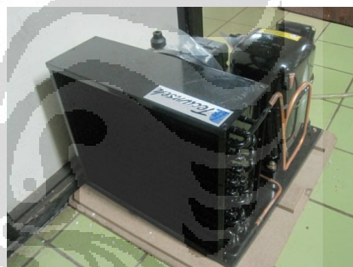
Gambar 3.3 Condensing unit High Stage Gambar 3.4 Condensing unit Low Stage
