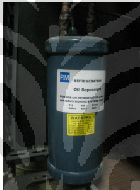
Gambar 3.10 Oil Separator
