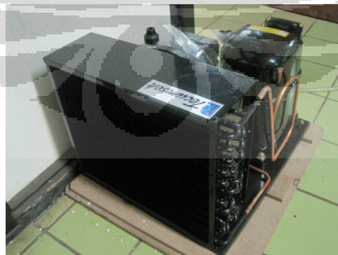
Gambar 3.4 Condensing unit Low Stage
