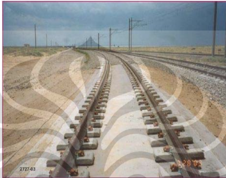
Figure 1. Independent Dual-Block Track (IDBT) at the demonstration site.
