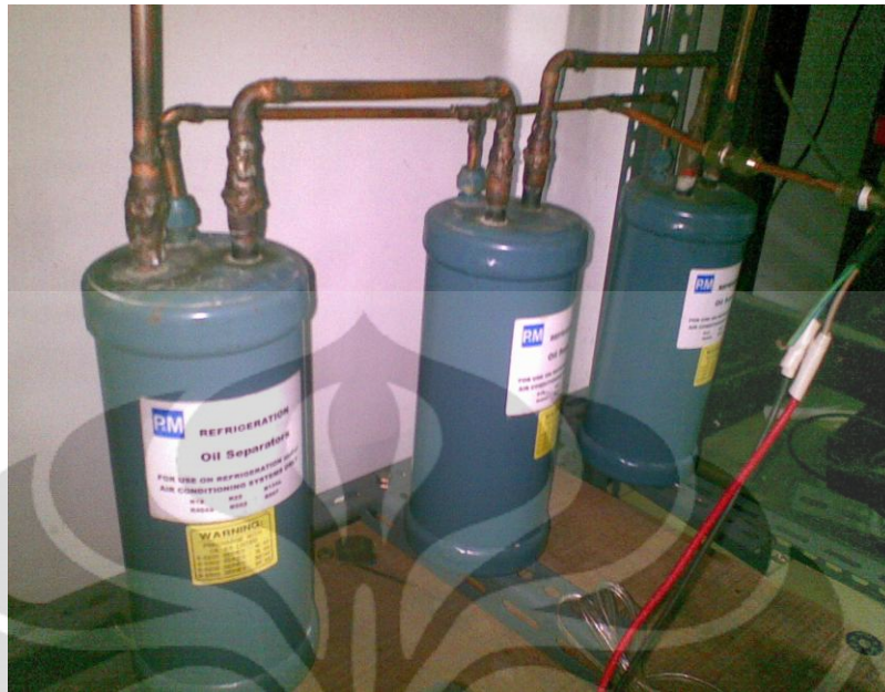
Gambar 3-8 Oil Separator
