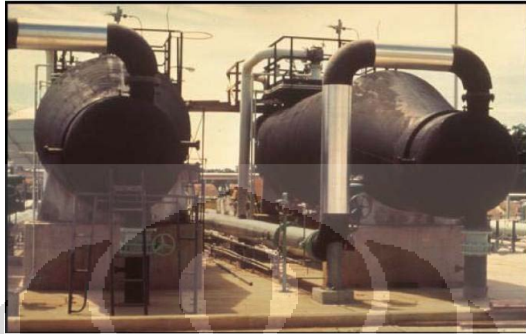
Gambar 2.9 Shell and Tube Vaporizers [5]
