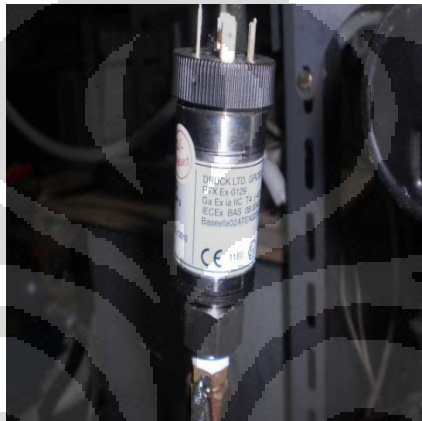
Gambar 4. 10 Pressure Transmitter
