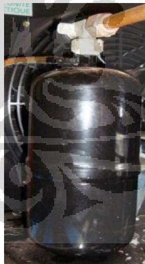
Gambar 3.7. Liquid Receiver
