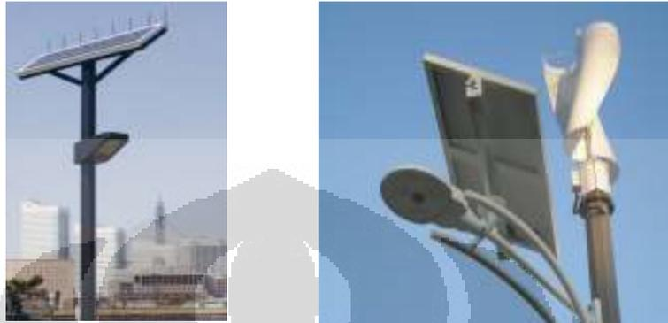
Gambar II.9 Sistem *Off-grid non domestic*
