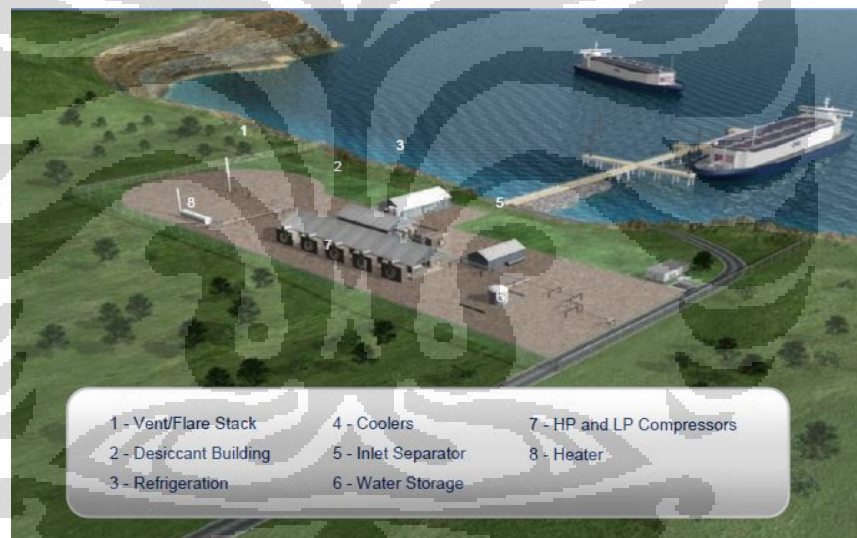
Gambar 4.2. Tipikal Terminal Loading CNG [10]
