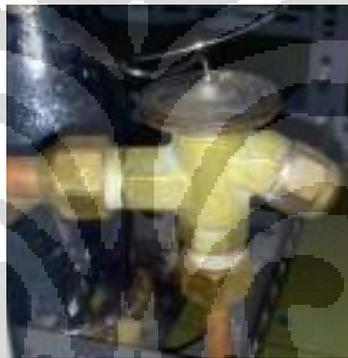
Gambar 3.13. Thermostatic Expansion Valve
