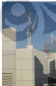
Gambar 4.29. Turby triple blade wind turbine design on top of a building [39]
