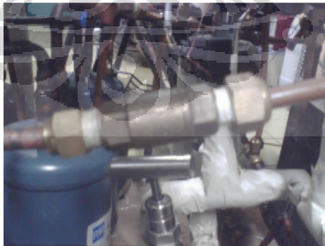
Gambar 3.11 Check Valve
