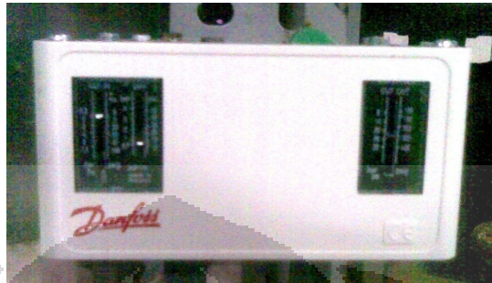
Gambar 3. 2 Hi-lo pressure control merk Danfoss.
