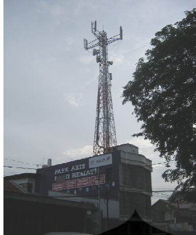
Gambar 2.4 Tower SST Rooftop
