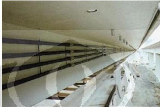
Gambar 2.1 External Post-tensioning
