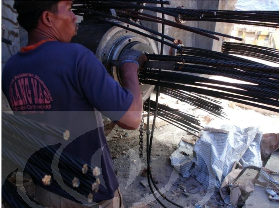
Gambar 6.7 Delivery Stressing Installation PC-U Girder
