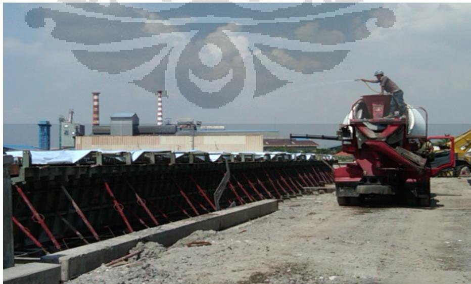
Gambar 5.5 Proses Curing
