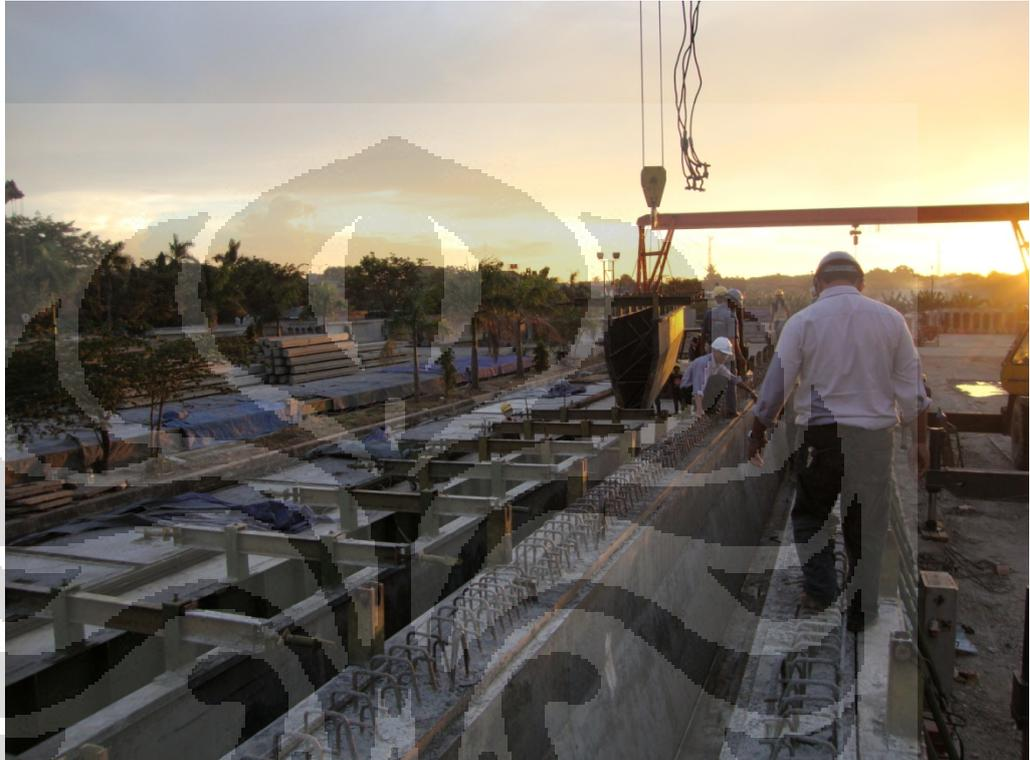
Gambar 5.6 Demoulding PC-U girder
