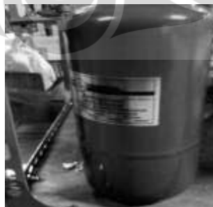
Gambar 3.9. Liquid receiver
