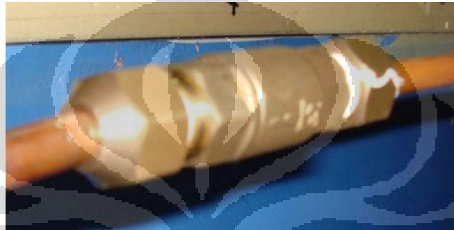
Gambar 3.13 Check Valve
