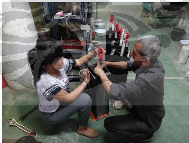
Gambar 4.4 Proses Pemasangan Vibrating Wire Embeded Strain Gauge
