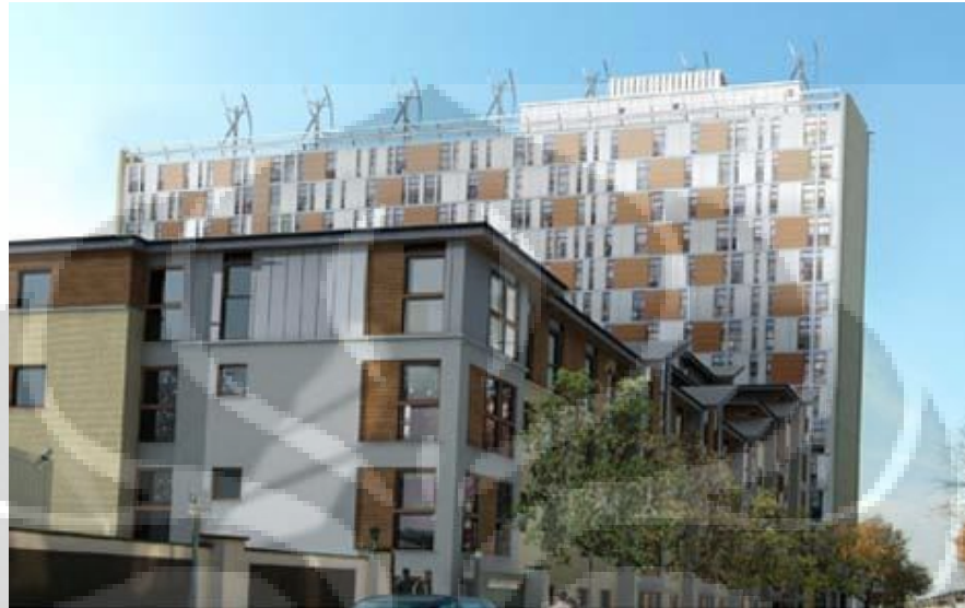
Gbr.4.12. City House di Croydon dengan 8 Turbin qr5 di atapnya (Sumber : http://www.vebra.com/vebra/buying/directory/London/Norwood )
