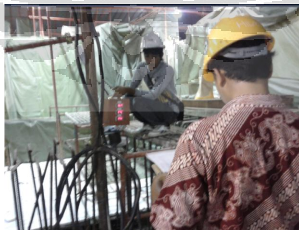
Pengukuran temperatur raft foundation
