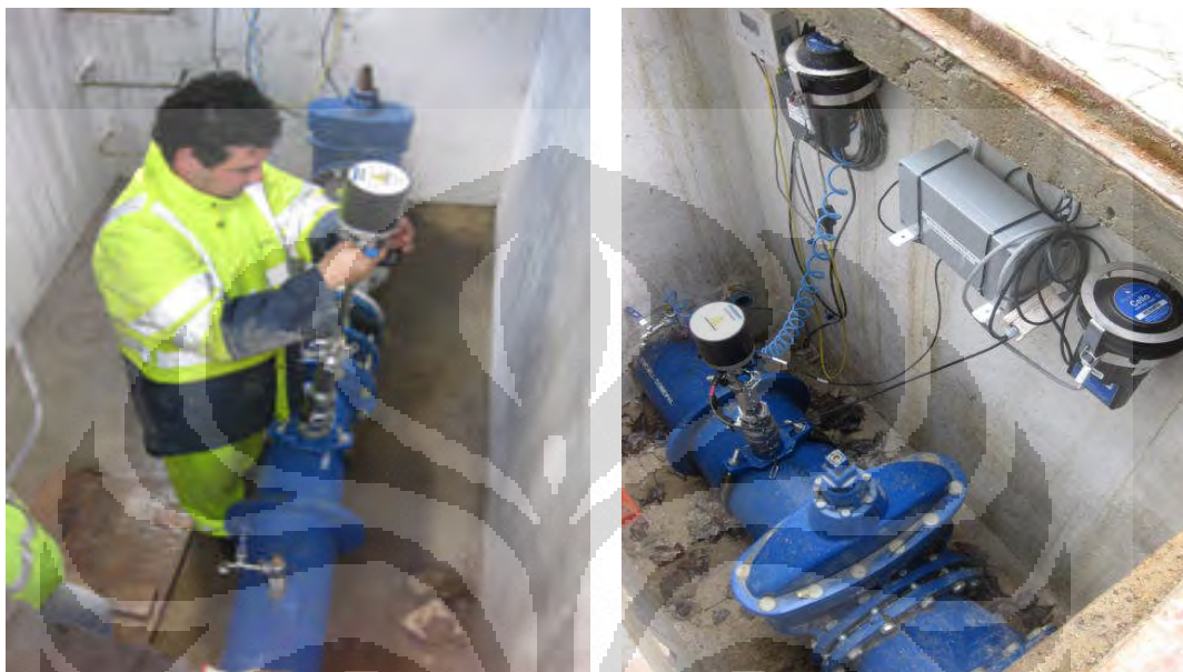
Figure 4.5 Implantation of Intellisonde™ in Lisbon water supply
