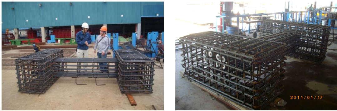
Figure 4.5 Typical reinforcement cage (a) Square hoops column; (b) Multi-spiral hoop column
