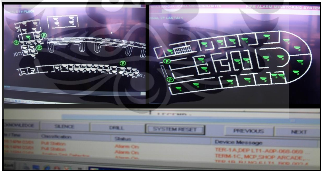
Gambar 6.8: Status Signal Fire Protection alarm dan detektor
