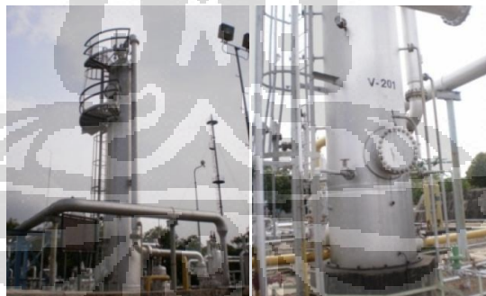
Gambar 6.8 Dehydration Contactor V-201 SP Pasir Jadi
