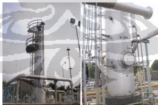
Dehydration Contactor SP PSJ
