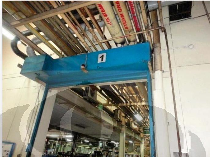
Gambar 6.11 Pintu Tahan Api di *Factory I*, PT. Bridgestone Tire Indonesia
