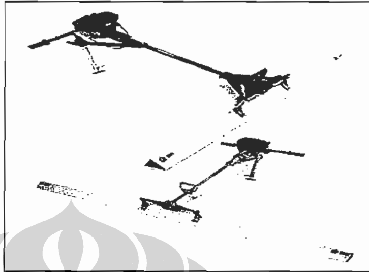
Gambar 7.2 – Concrete screeding
