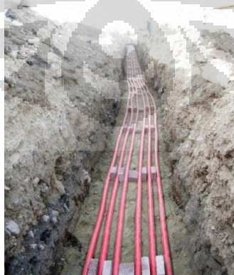
Gambar 2.3. Underground cables
