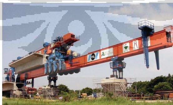
Gambar 2.9 Metode Launching Carrier Full Span
