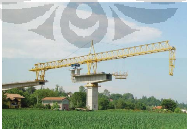
Gambar 2.7 Metode Balanced Cantilever
