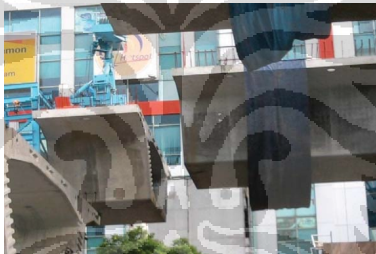
Gambar 3.9 Erection Girder
