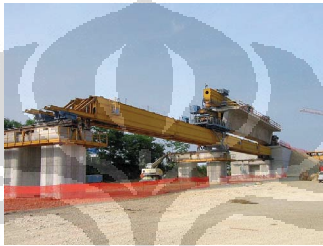
Gambar 2.8 Metode Launching Carrier
