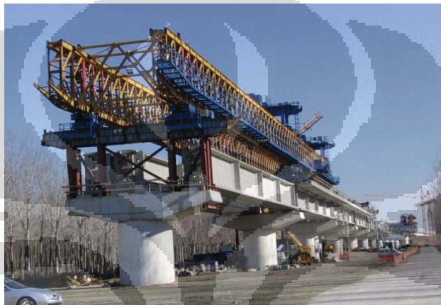
Gambar 2.6 Metode Span by Span
