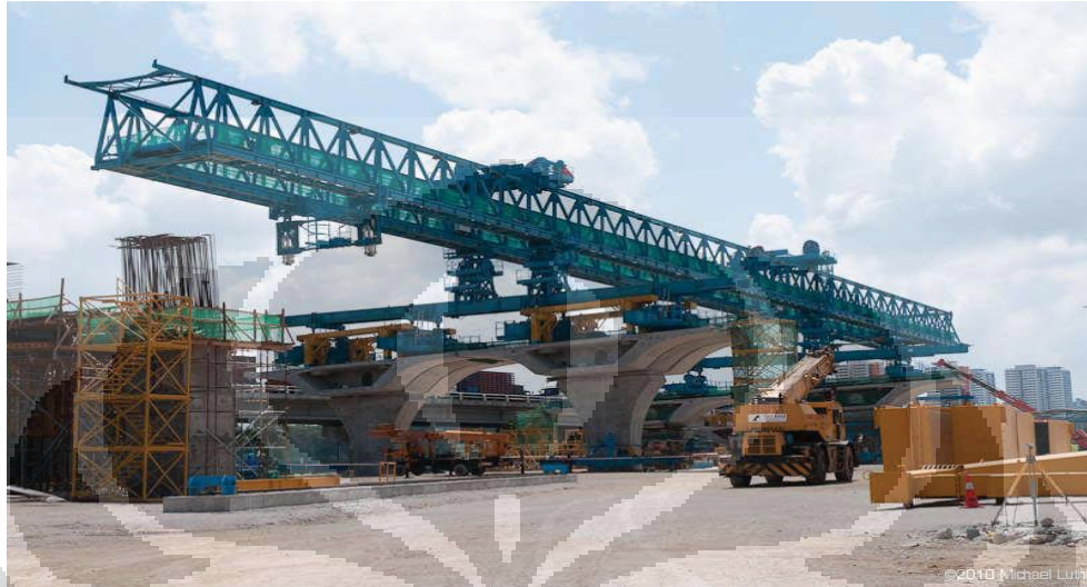
Gambar 3.4. Launcher Balanced Cantilever Gantry
