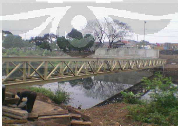
Gambar 2.5 Metode Launching Frame
